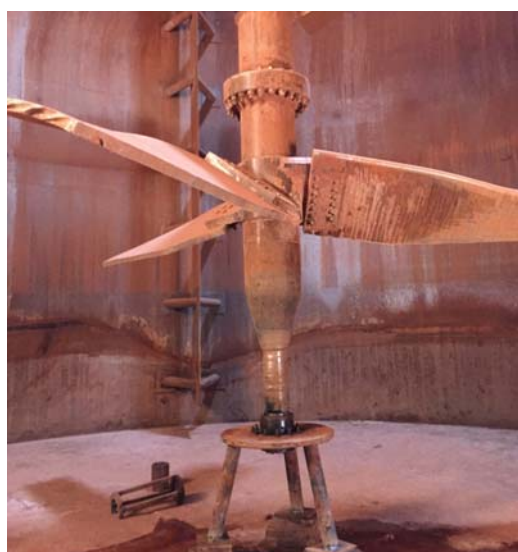
Figure 14. View inside a cleaned desilicator.
